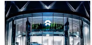
Chengdu NIO House
