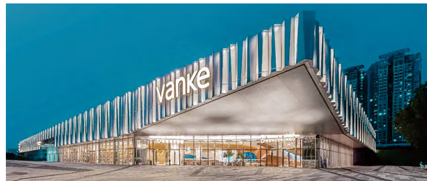
Vanke Huadiwan Life Center in Guangzhou
