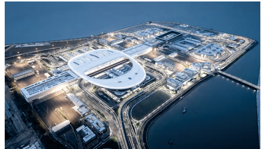
Hong Kong-Zhuhai-Macao Bridge
